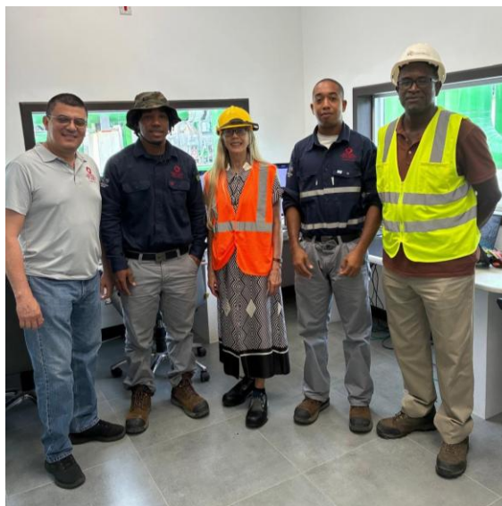
New Zealand High Commissioner, H.E. Linda Te Puni visited and met with staff and stakeholders at the 10 MW Geothermal Power plant in Roseau Valley, Dominica.
