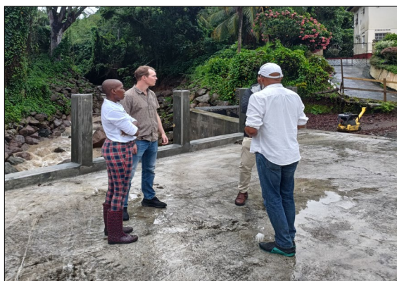
Figure 3: Assessing road and infrastructure in Grenada with the Geothermal Project Management Unit
